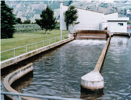
Fig. 4. Ongoing treatment, with FOG control.
